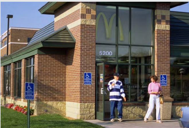
Individually designed free-standing franchise use.
