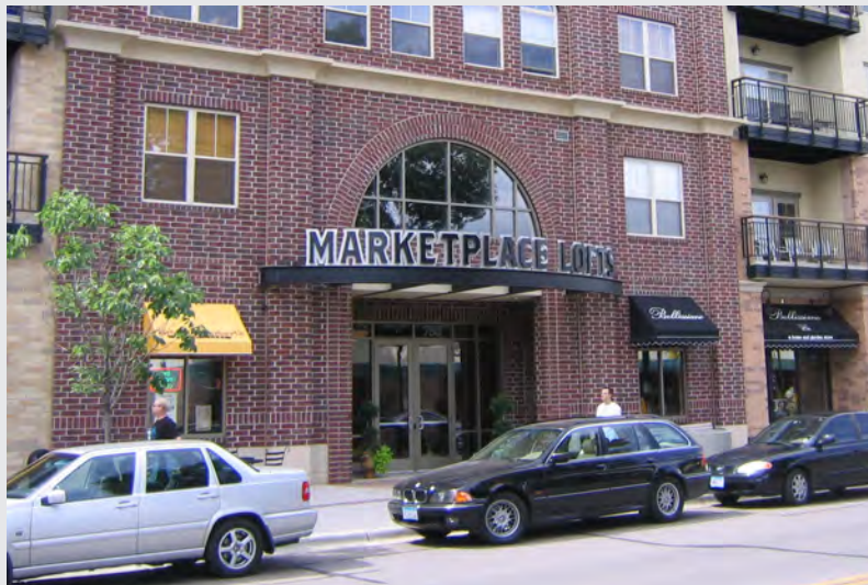
Recessed entry with canopy and sign.
