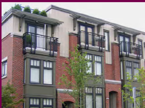
Flat roofed building with varying roof heights.
