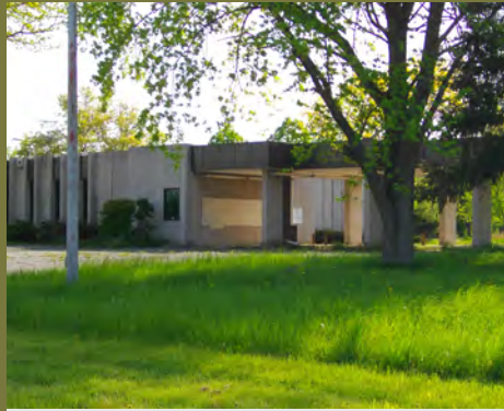
Vacant bank building at the southeast corner of the district
