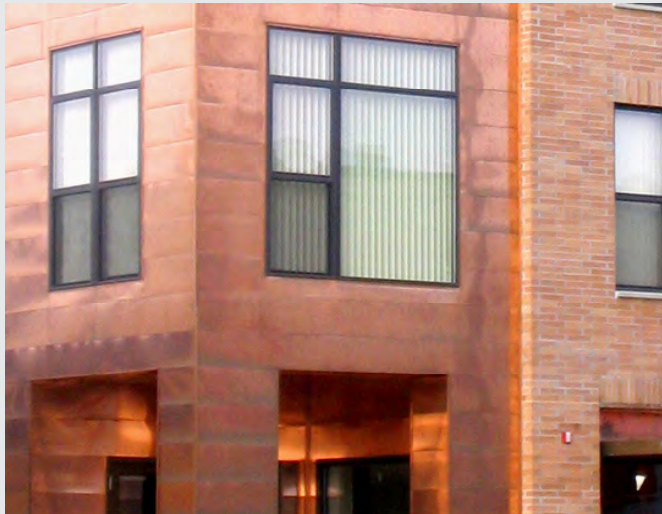
Copper siding and brick
