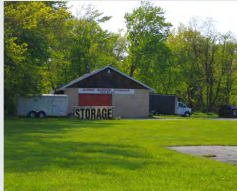
Existing mini storage facility.
